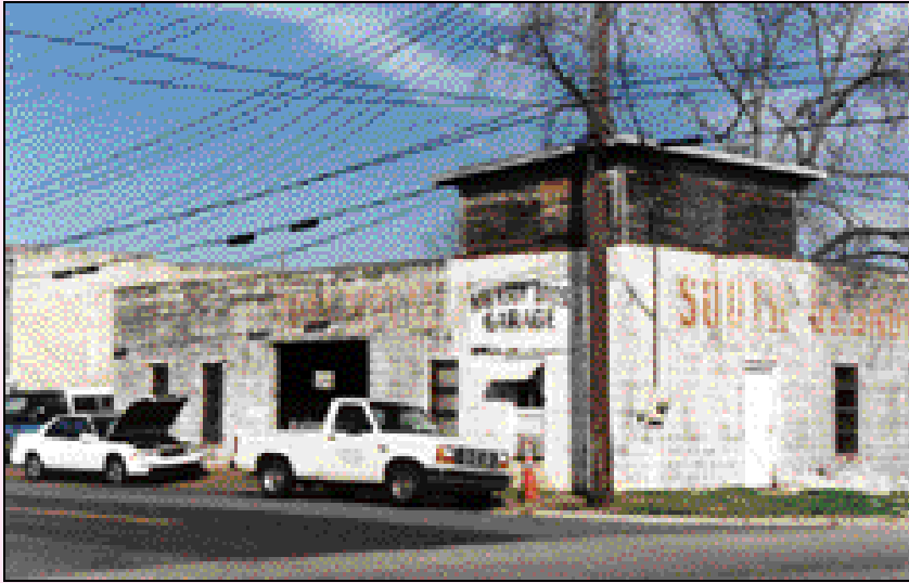
Robinson Brothers Garage constructed with cast-concrete blocks.
