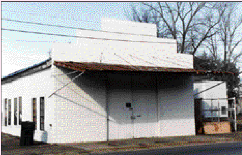
Moultrie Machinery and Foundry Company constructed by 1912 with a cast-concrete block front facade.
